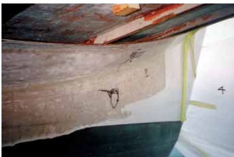
Insufficient wing deck beams made of unsuitable cedar
