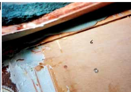
Shoddy workmanship inside a locker
